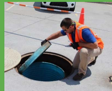
Inspecting a containment sump
